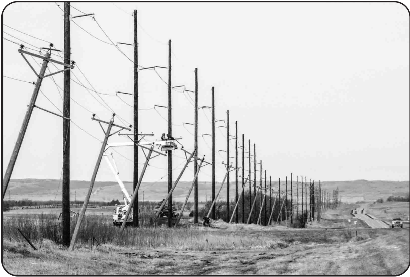
A 2021 telephoto view of Highway 11 near Pheasant Lake illustrates the workaround procedures needed to install the new, modern line in the same path as the older line. Earth around each of the old poles was dug up and the poles tilted to keep the existing, live lines in service while the new poles went up and the new highline wires strung. The highline runs all the way from Leola, South Dakota to the massive substation west of Ellendale that was completed in 2018 (photo by Ken Smith April 2021)
