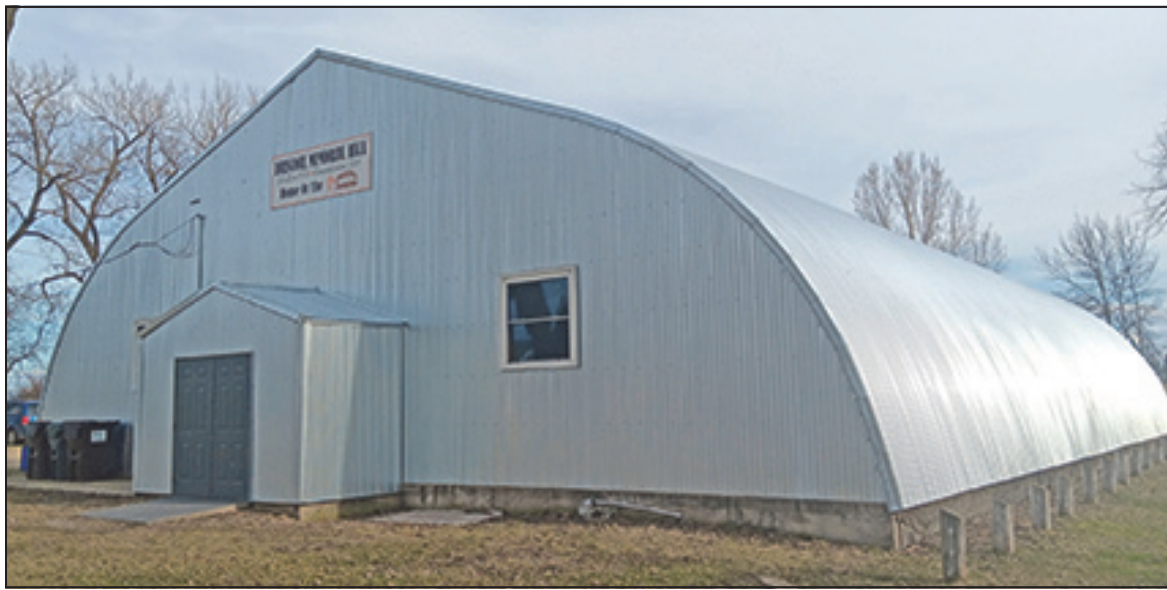
The front of the newly renovated Driscoll Hall. (More pictures on page 16)
