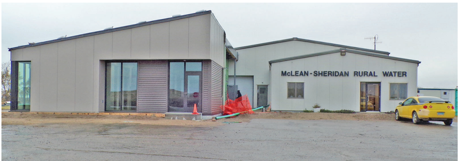
McLean Sheridan Rural Water District plant under construction.
