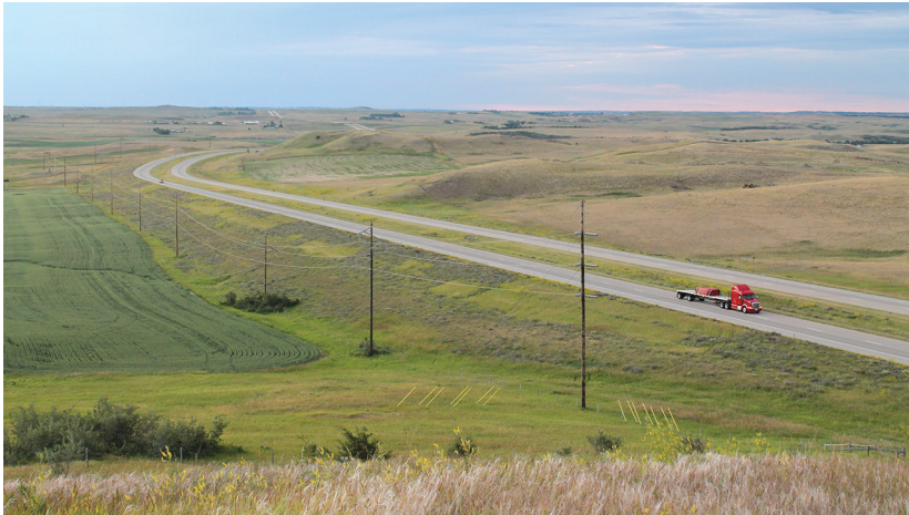
I-94 Schlosser Pass Lat 46 51 54 Long 101 11 40, July 3 2017, looking east.
