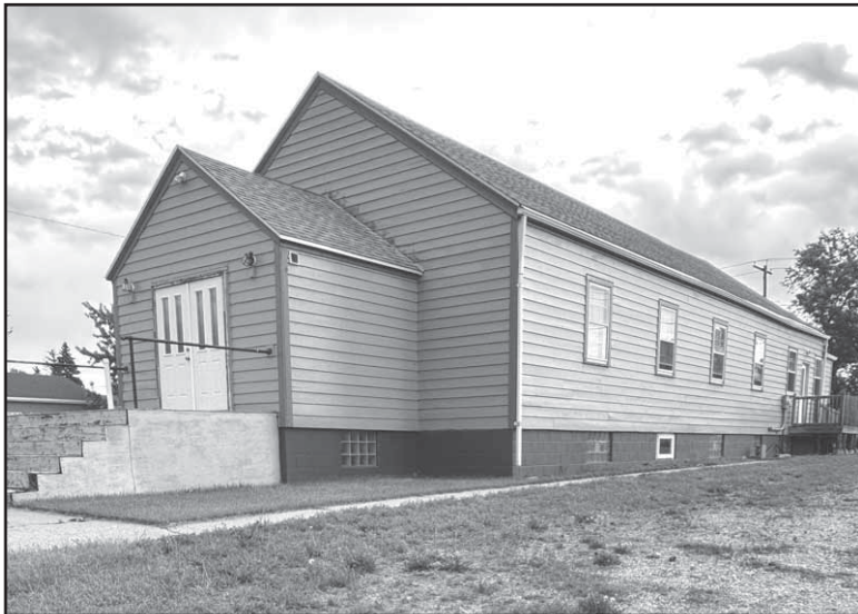
The big, blue building on Trooper Ave. is set to debut as Garrison's new community center and meeting space next month. (Tyson Matthews)
