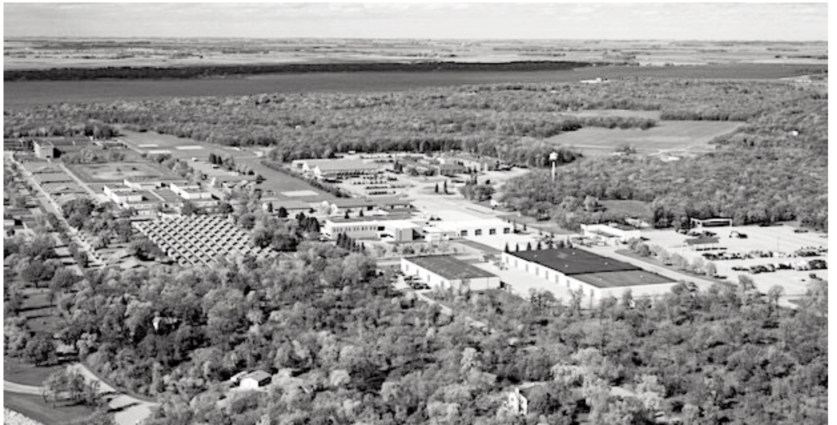
Camp Grafton, a National Guard facility near Devils Lake, North Dakota. (Courtesy of North Dakota National Guard)
