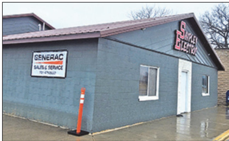
Shipley Electric is located on Highway 3 in Dawson
